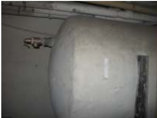
HOMOGENEOUS AREA # 25 TSI – HOT WATER TANK
