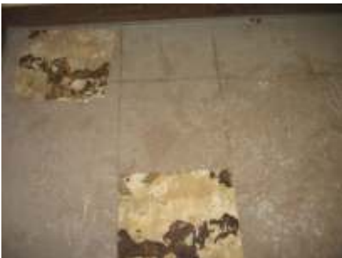
HOMOGENEOUS AREAS # 18, 19 12" VINYL FLOOR TILE (BROWN)/ADHESIVE
