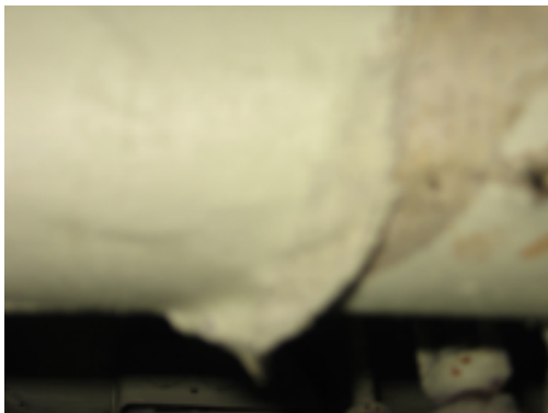
HOMOGENEOUS AREA # 27 TSI PIPE CLOTH
