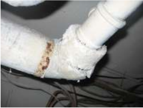
HOMOGENEOUS AREA # 29 TSI PIPE ELBOW
