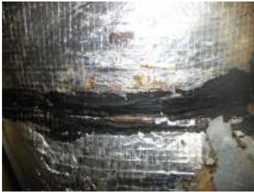
HOMOGENEOUS AREA # 37 HVAC DUCT ADHESIVE (BLACK)
