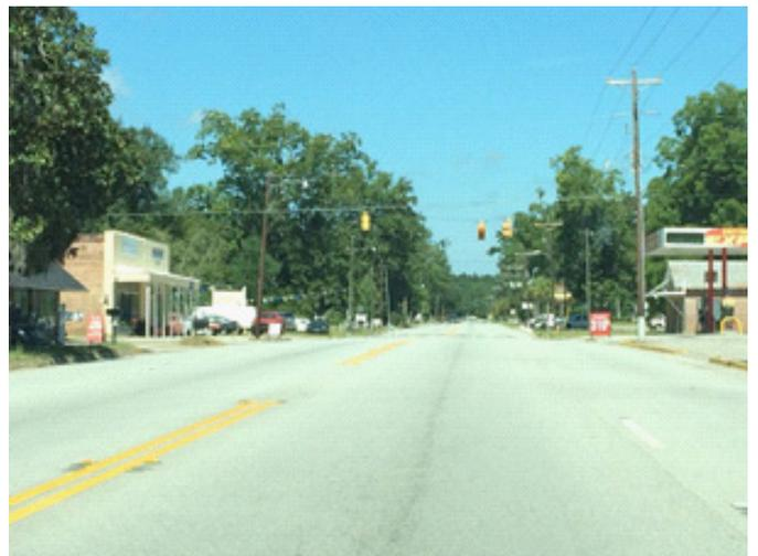
**Roadway design doesn't typically change to account for potential non-motorized traffic through population centers in Colleton County.** For example, the roadway pictured is wide to cross and only has sidewalks on one side. This type of design is unsafe and discouraging to bicycle and pedestrian traffic. (location: Alternate 17, Cottageville)
